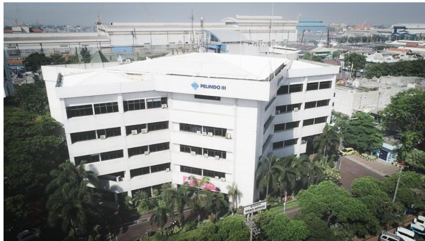
Gambar 1. Foto Gedung A PT. Pelindo Regional III
